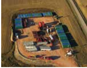
Hydraulic Fracturing Spread
